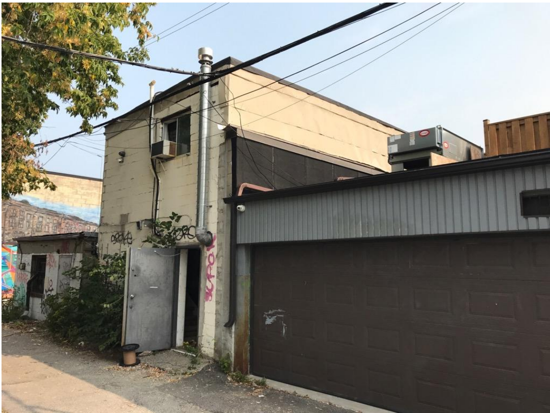
Figure 7 View from lane looking east toward building
