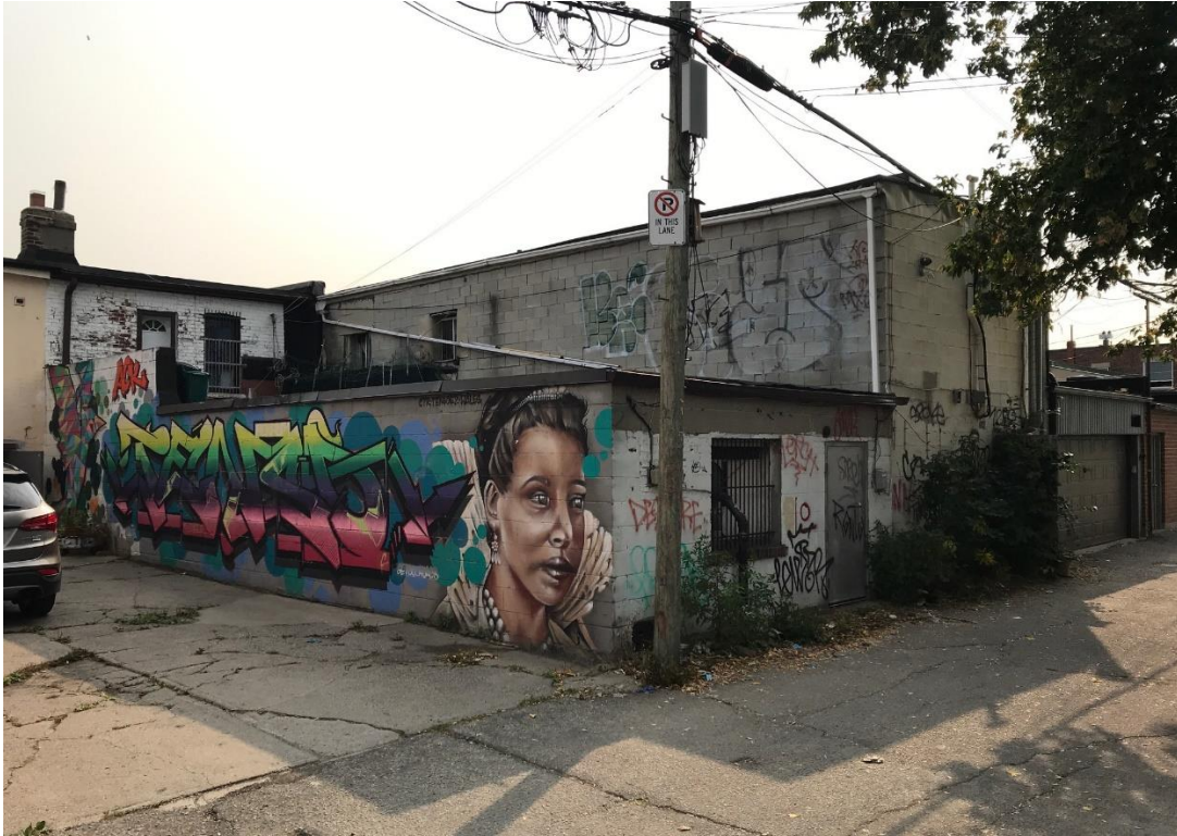
Figure 6 View from lane looking west toward building
