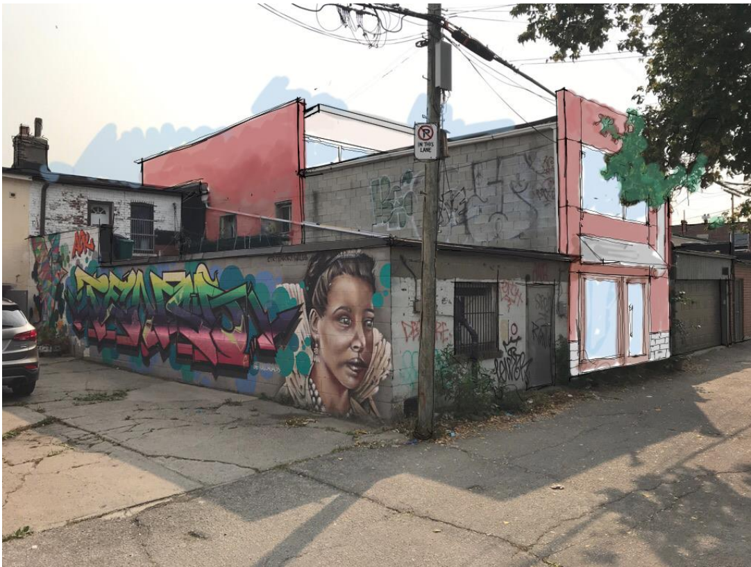
View from lane showing new third floor and new back wall
