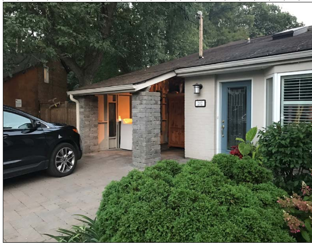
VIEW TOWARD EXISTING HOUSE SHOWING AREA OF NEW WORK
