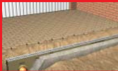
4. Push-fit grates into channels. Protect with plastic if using concrete or asphalt paving.
