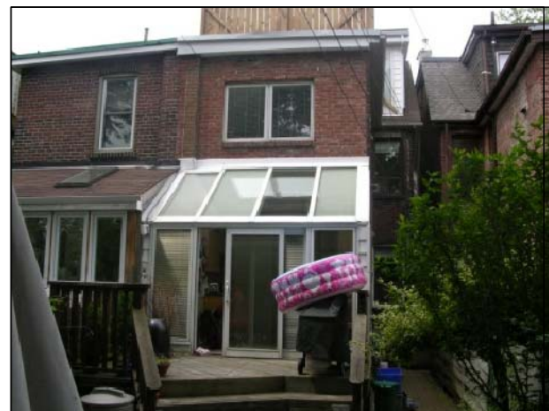
2 EXISTING HOUSE FROM REAR A1 Scale: NTS
